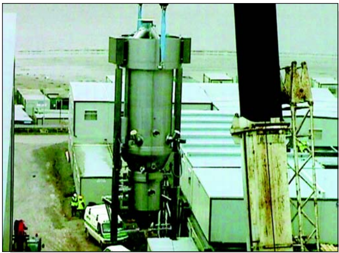
Figure 4. Example equipment being installed.
